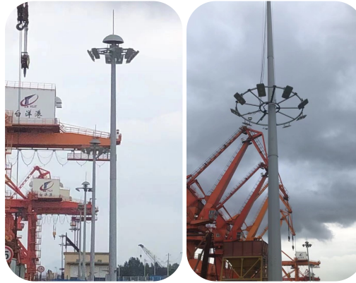
Shanghai Port Group Baiyang Wharf
